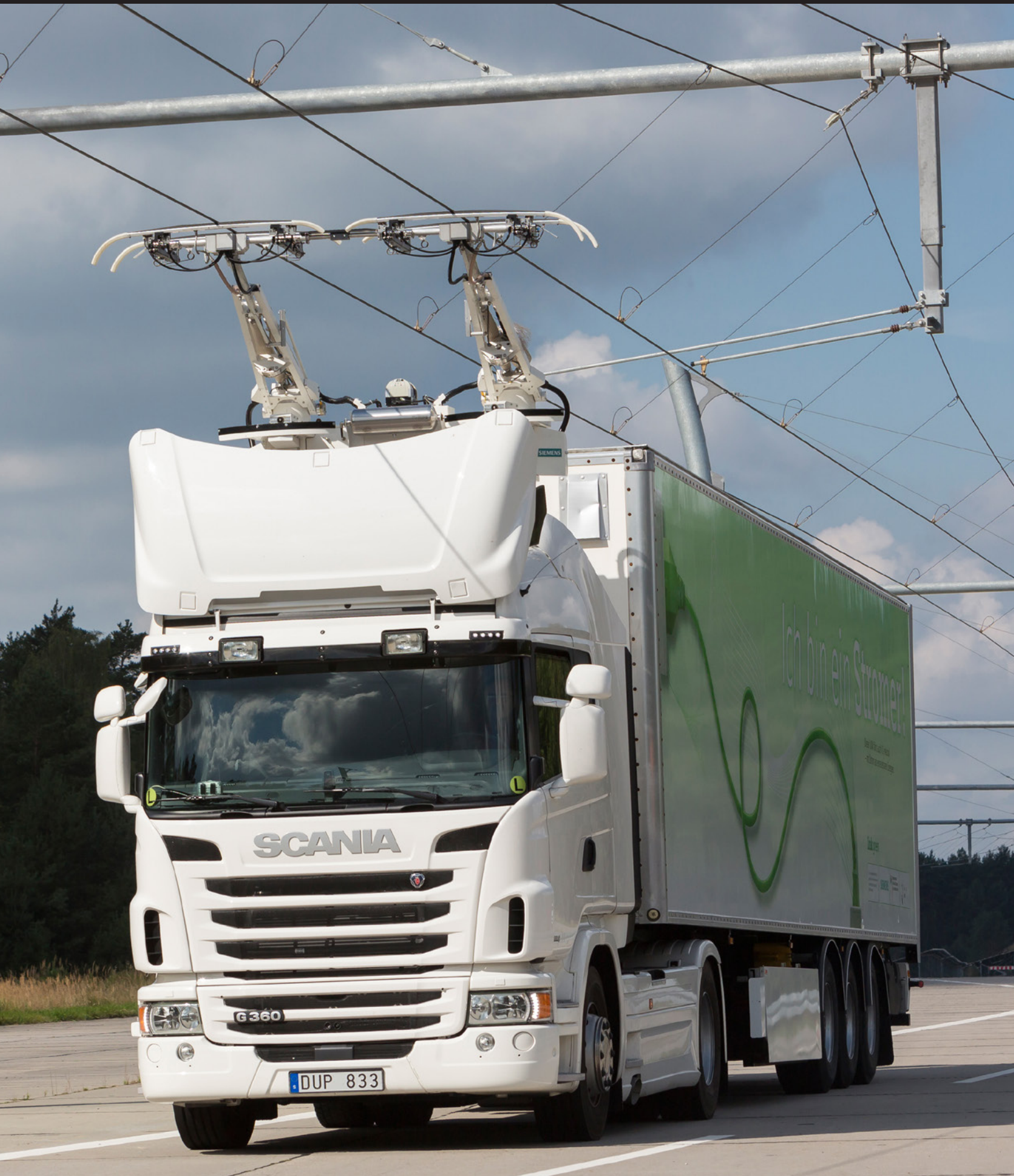
SIEMENS' eHIGHWAY TEST TRACK - GROSS DÖLLN, GERMANY
